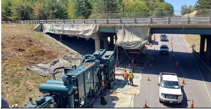
Type 1- Interstate Bridge - Interstate roadway is open over Local Road - Equipment on local road- clears out daily
