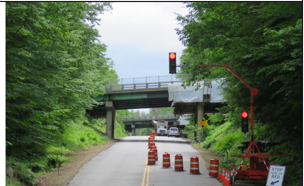
Type 2- Interstate Bridge - Interstate roadway is open over Local Road - Equipment on local road - stays 24/7 (w traffic signals)
