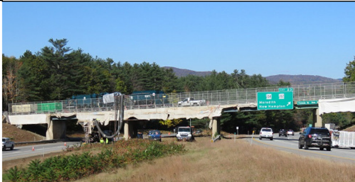
Type 3- Local Road Bridge - Equipment on bridge - stays 24/7 (w barrier, barrels, or traffic signals) over Interstate - Rapid deployment unit on Interstate - clears out daily
