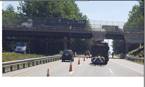
Type 3- Local Road Bridge - Equipment on bridge - stays 24/7 (w barrier, barrels, or traffic signals) over Interstate - Rapid deployment unit on Interstate - clears out daily
