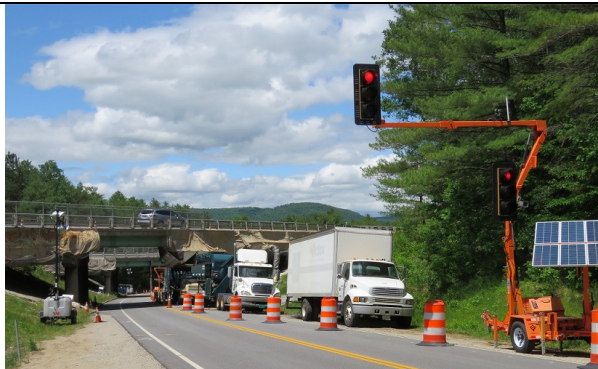
Type 2- Interstate Bridge - Interstate roadway is open over Local Road - Equipment on local road - stays 24/7 (w traffic signals)
