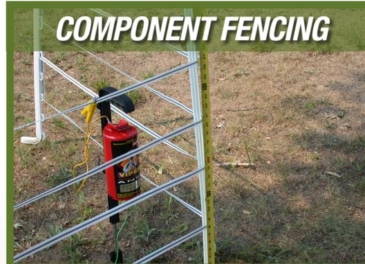
*A component fence system can be used around existing buildings and poultry runs. Constructed with tread-in posts or nail-on screw-in insulators, it includes four strands of electrified conductor at 8"-10" intervals for bears. Bottom strands can be 4"-6" for smaller predators.*
