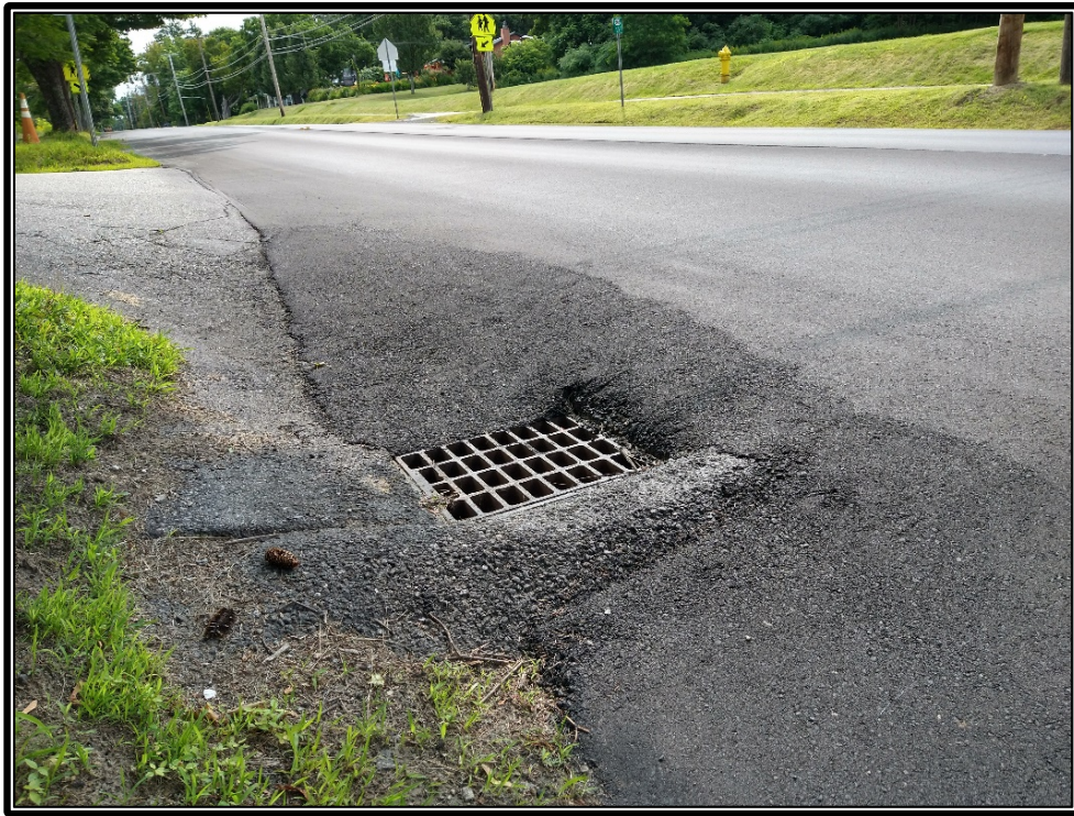
Photo 5: Vertical drop-off at existing drainage grates
