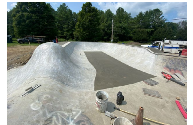
Second Phase in Construction
