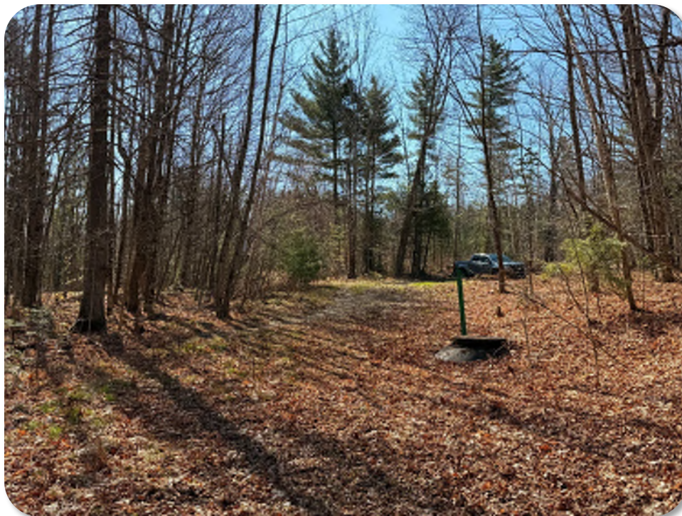
Photo 3: Looking east towards Maplewood Hill Road at Cross Country Sewer.
