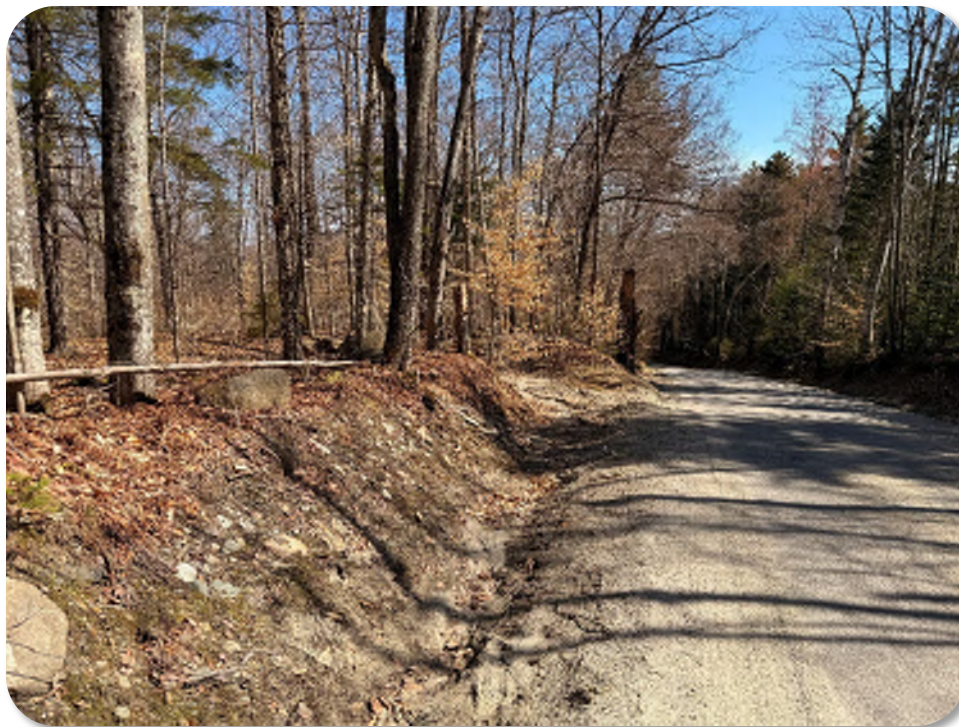
Photo 5: View of roadside ditch turnouts.
