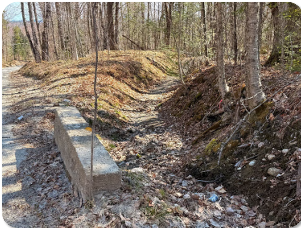
Photo 7: Existing culvert head wall and drainage ditch on the east side of Maplewood Hill Road.
