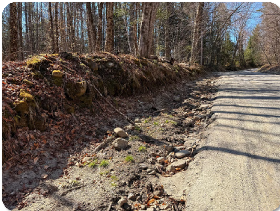
Photo 10: Looking south at roadside ditching along Maplewood Hill Road.
